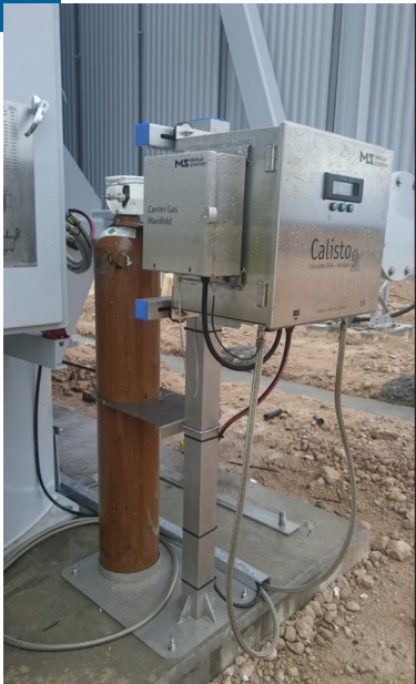
Solar farm at South Africa
